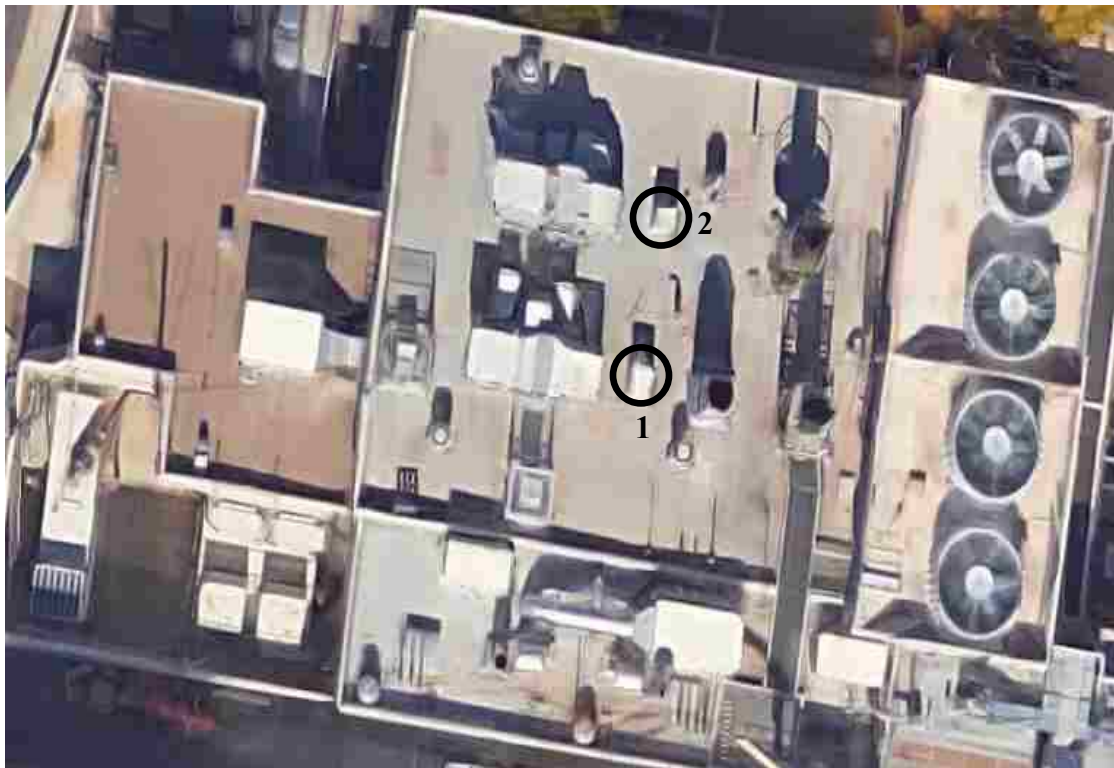
Fig. 8.5. Google image of the roof of Ford Utility Center.
